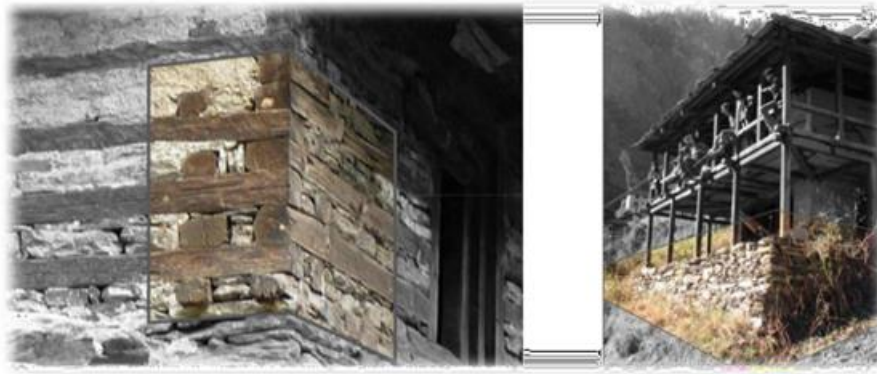
Figure 10 Kath khuni wood structure, gaps to be filled with stone/rubble
