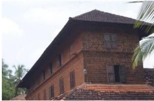
Figure 30 Exposed stone masonry
