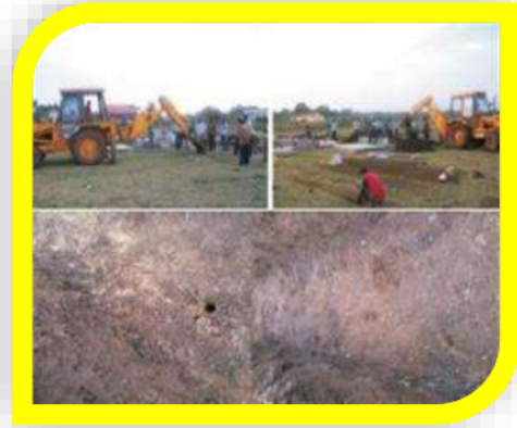
Day 1- Marking of foundation, Earth work excavation by Back Hoe Excavator
