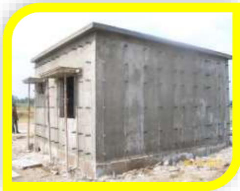
Day 4: De-shuttering of wall & roof, curing compound application, filling the holes
