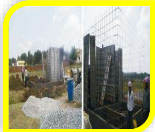
Day 2: Sand Piling and Sand Bed filling, Steel fabrication for Foundation & Plinth Beam, Concreting of Foundation & Plinth Beam, fabrication of steel for wall & roof
