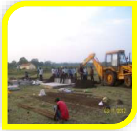
Day 1- Marking of foundation, Earth work excavation by Back Hoe Excavator
