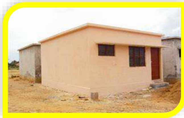
Day 5: Doors & Windows fitting, Sanitary & electrical fittings, Whitewashing /colouring, flooring, finishing
