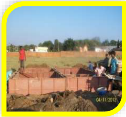
Day 2: Sand Piling and Sand Bed filling, Steel fabrication for Foundation & Plinth Beam, Concreting of Foundation & Plinth Beam, fabrication of steel for wall & roof
