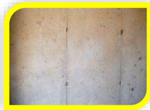
Day 4: De-shuttering of wall & roof, curing compound application, filling the holes
