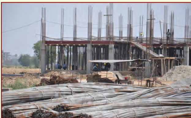
Construction of CDTS building in progress
