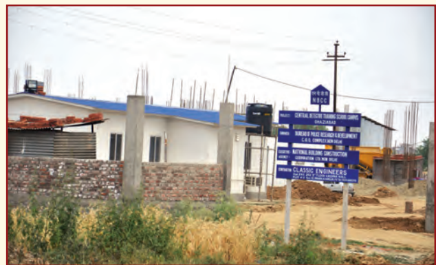
A view of construction site on the allotted land for CDTS
