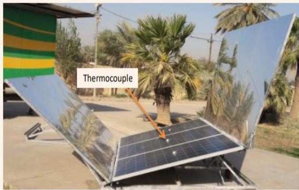
Figure 1. PV panel under sunlight reflection
