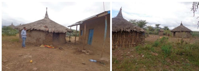
Figure 3. Showing roof top rain water harvesting practice in the study area.
