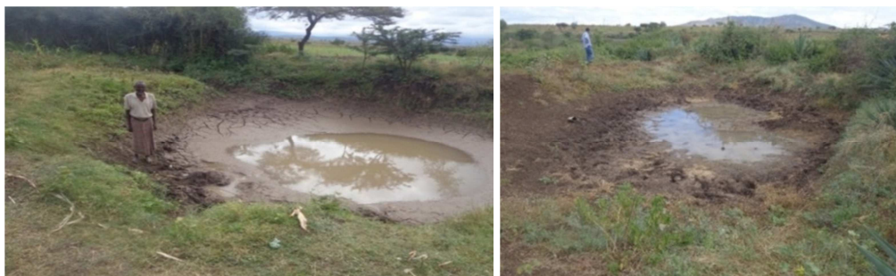
Figure 5. Traditional RWH technology (Kure) at Hamaressa kebele farmer's farm land.
