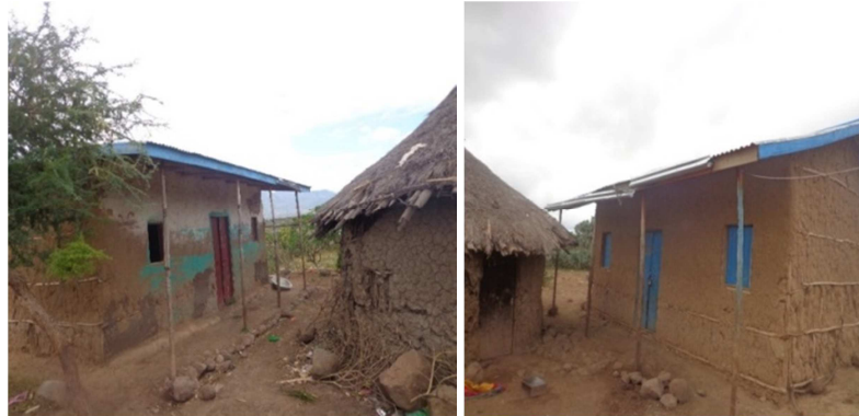
Figure 4. Showing roof top rain water harvesting practice in the study area.
